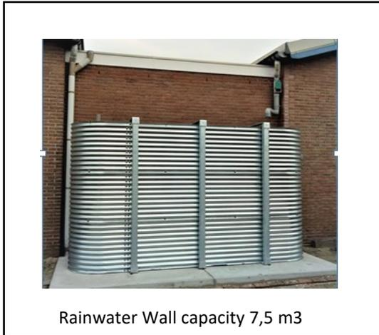
Rainwater Wall capacity 7,5 m3
