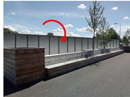
*Picture. 4: Rainwater Wall, total volume 60 m<sup>3</sup>*
