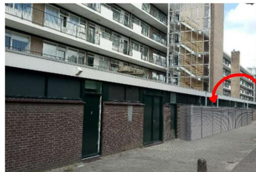
Picture 2: Rainwater Wall, total volume 25 m<sup>3</sup>
