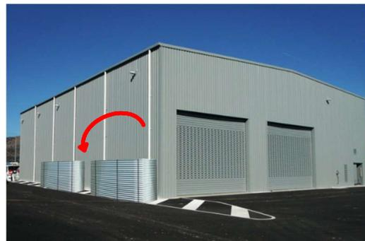
Picture 1: Rainwater Wall, total volume 16 m<sup>3</sup>
